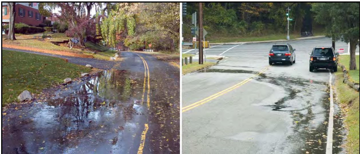
Figure 1-3. Examples of Drainage Issues
