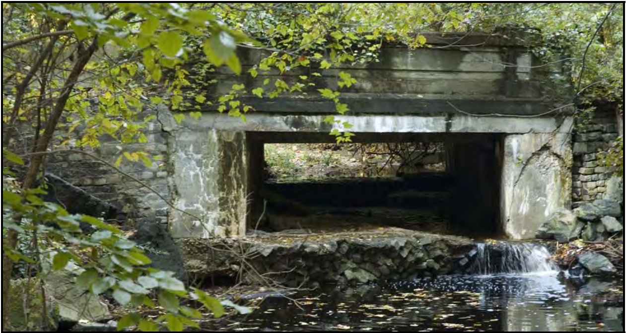
Figure 1-4. Pinehurst Run Culvert
