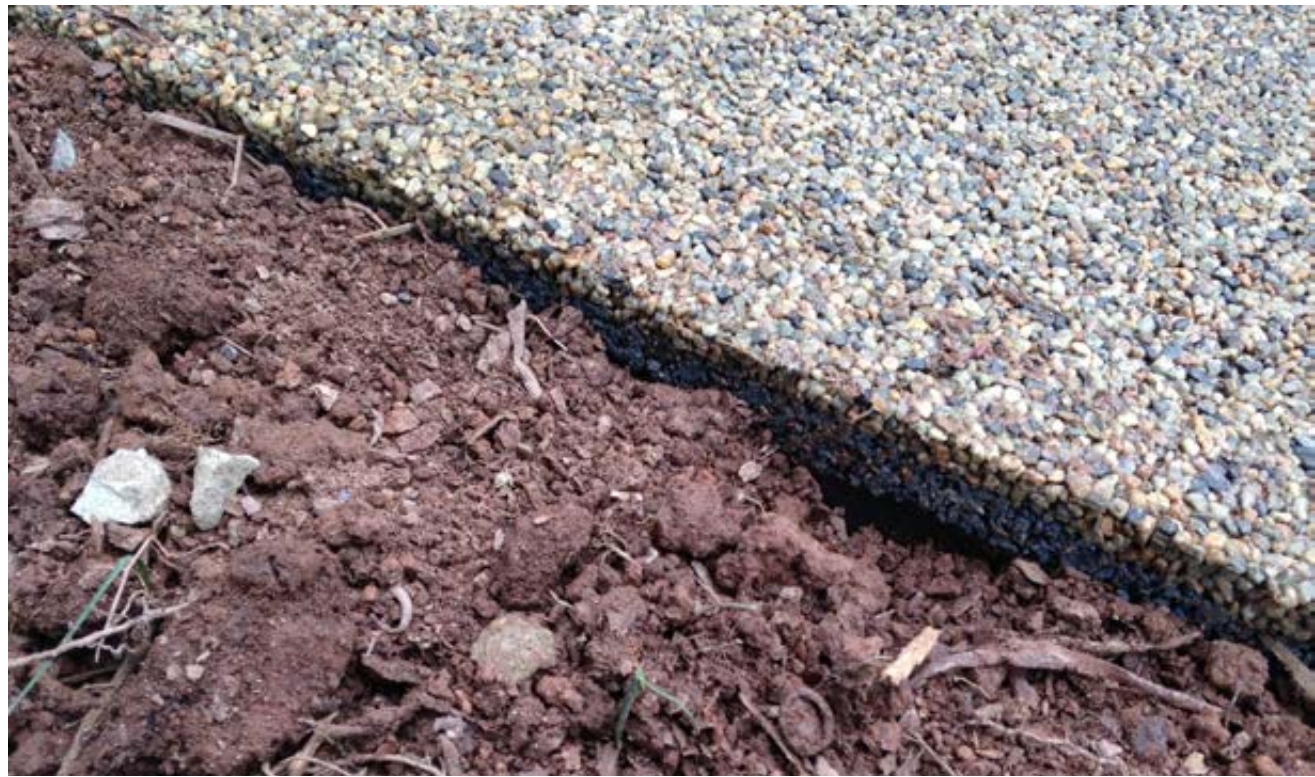
Surface to replicate exposed aggregate pavement
