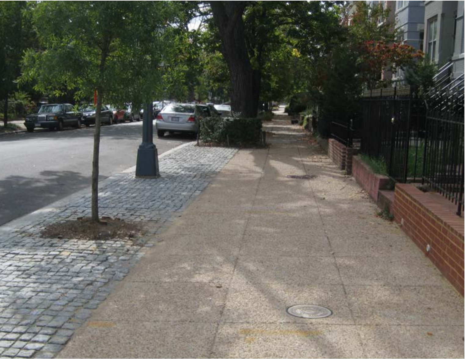
Exposed aggregate concrete is commonly used in residential sidewalks in lieu of regular concrete to better blend in with the surrounding natural or built environment.
