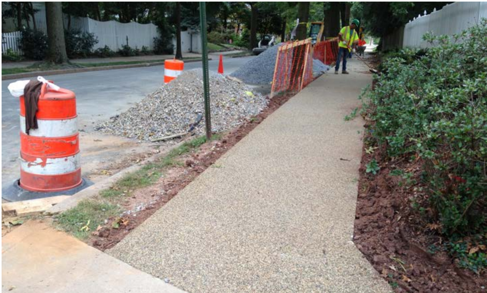
Pervious sidewalk installation nearby in RiverSmart Washington
