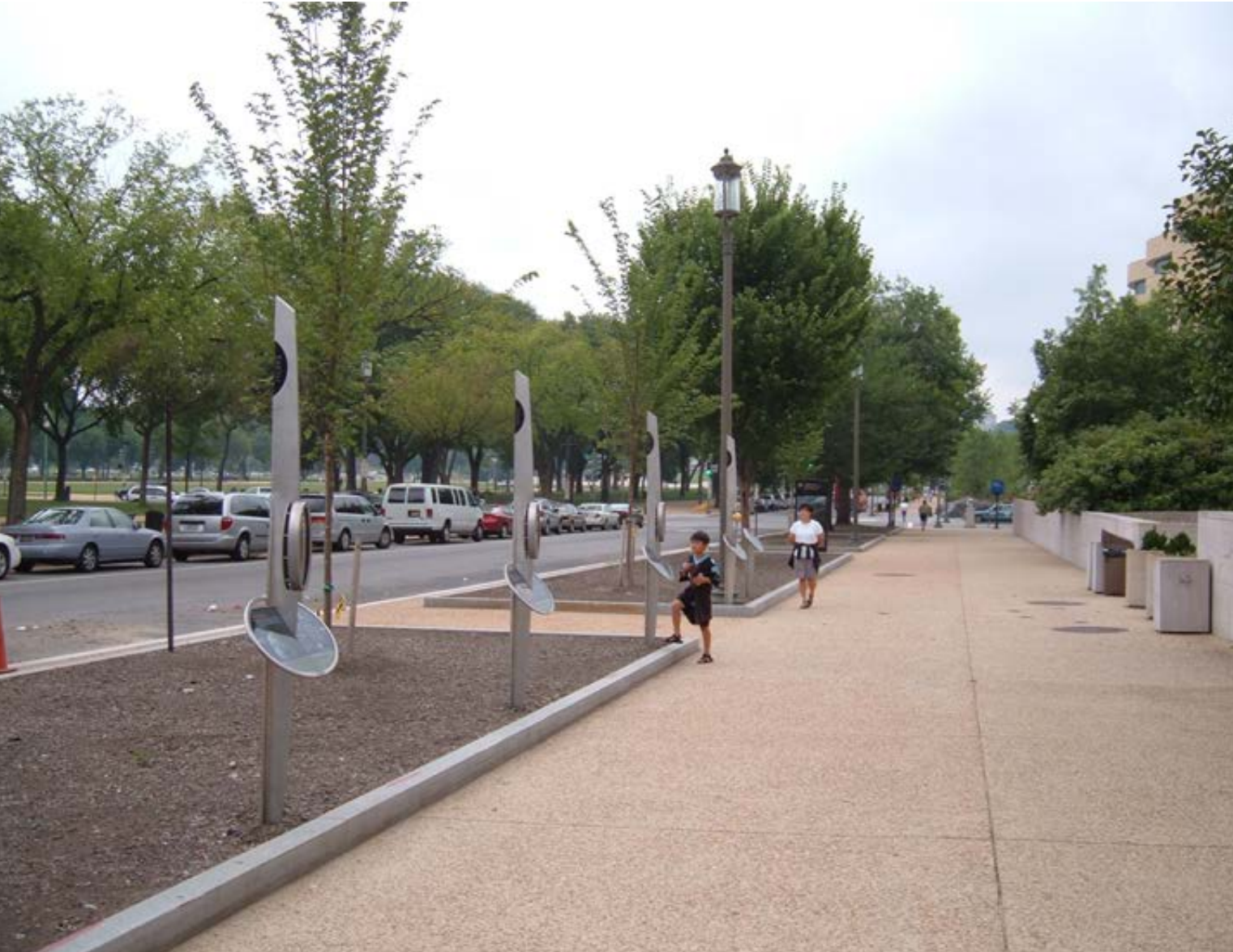
Exposed aggregate concrete is used throughout the National Mall to blend in with the nearby loose stone walkways and other surrounding areas.
