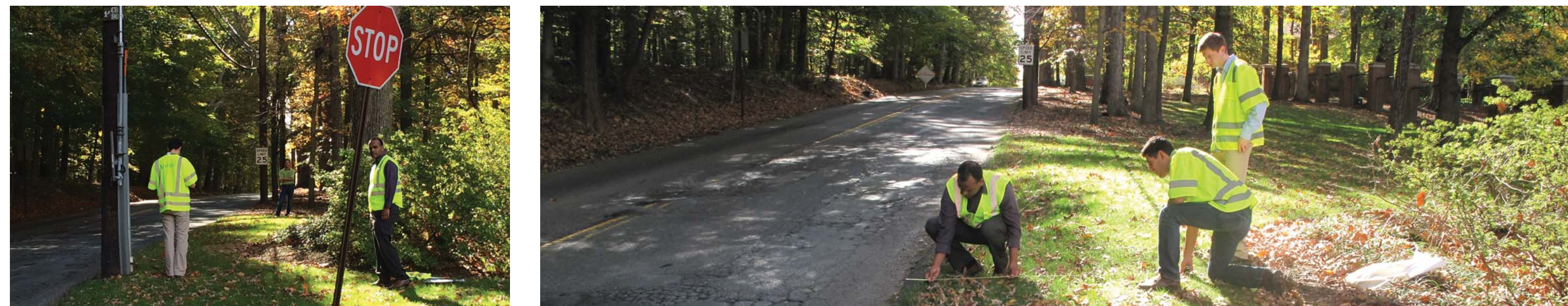
Using string and measuring tools, we laid out a sidewalk path in front of Chatsworth / Unicorn Lane
